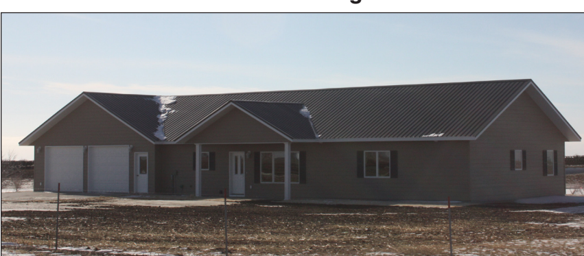
United Feeders manager's house
